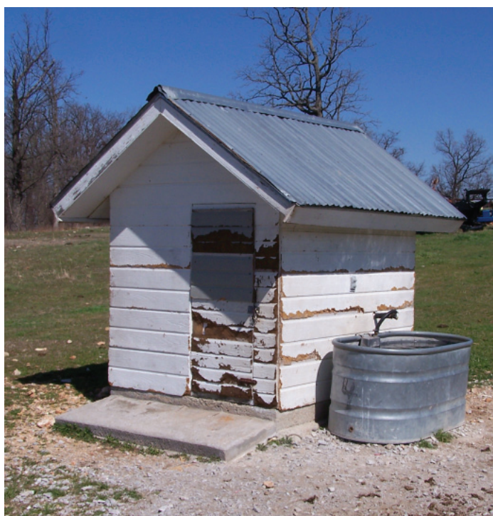
Figure 2. The well-house shaft is a 120-deep shaft used as a source of water for livestock today.
