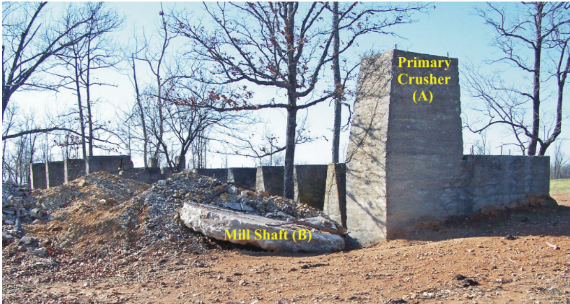
Figure 6. Foundation for the Log Cabin mill. The tallest pier (A) is where the primary crusher was located; and the mill shaft (B) was beneath the tilted concrete pad.
