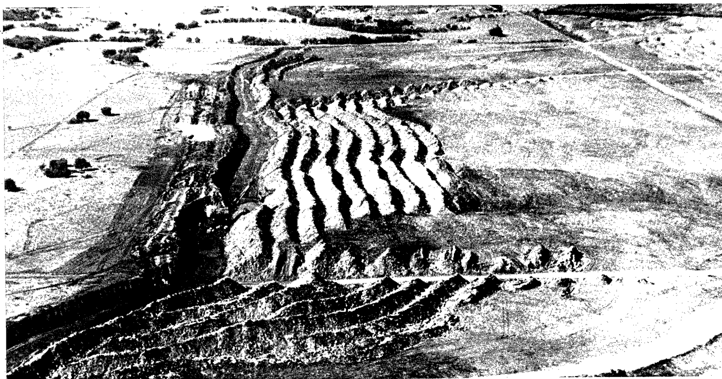
Figure 23. Photograph of strip mine in northeastern Rogers County, Oklahoma, 1971, showing, from left to right, undisturbed land underlain by measured reserves, a narrow belt drilled for shooting and overburden removal, mine pit with coal exposed, alternating furrows and ridges where coal has been mined and overburden piled, and reclaimed land that has been seeded (by helicopter) with grass. (Courtesy of K.S. Johnson.)
