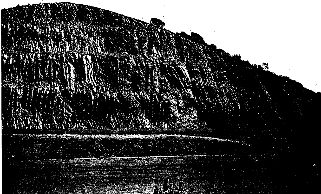
Figure 26. North flank of Arbuckle anticline, looking east on Interstate 35. Viola Limestone overturned above Bromide Formation; contact at station 2658 + 60 feet. Strike, N. 55^{\circ} W.; dip, 75^{\circ} SW. Contact between Pooleville Limestone Member and Mountain Lake Member (at right) of Bromide Formation is at station 2657 + 40 feet. This cut is deepest in Arbuckle Mountains, with a vertical span of 156 feet.
