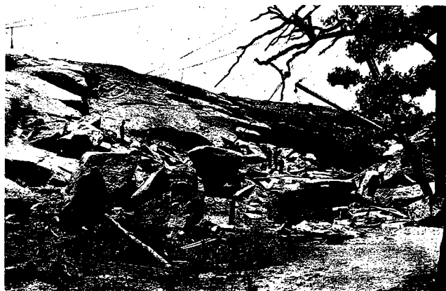
Figure 43. Stop 6. Capitol quarry at Ten Acre Rock. Photograph was taken in 1916, when Tishomingo Granite of Precambrian age was being quarried as a source of dimension stone for use in construction of state capitol at Oklahoma City. Quarry appears much the same today, not having been actively worked in the intervening years, except that original equipment has been removed.
