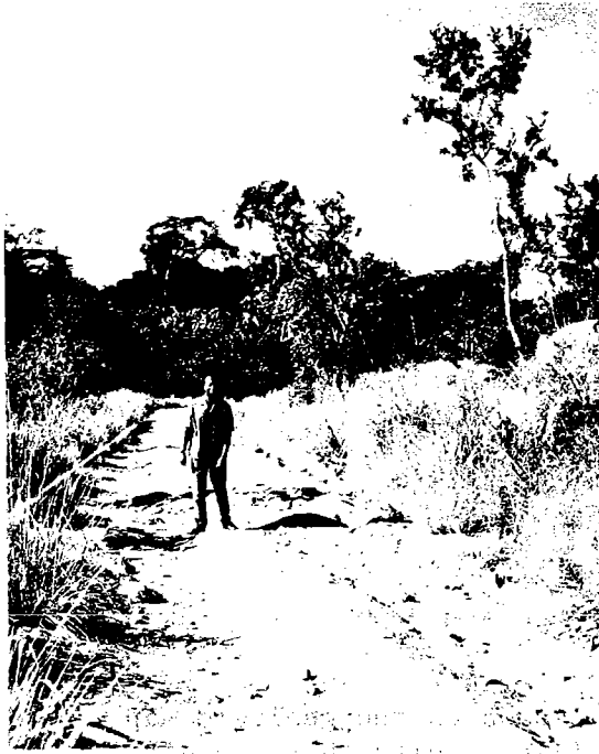
Figure 5. A section of road developed in weathered clayey and bouldery soil of the Crystalline rocks.
