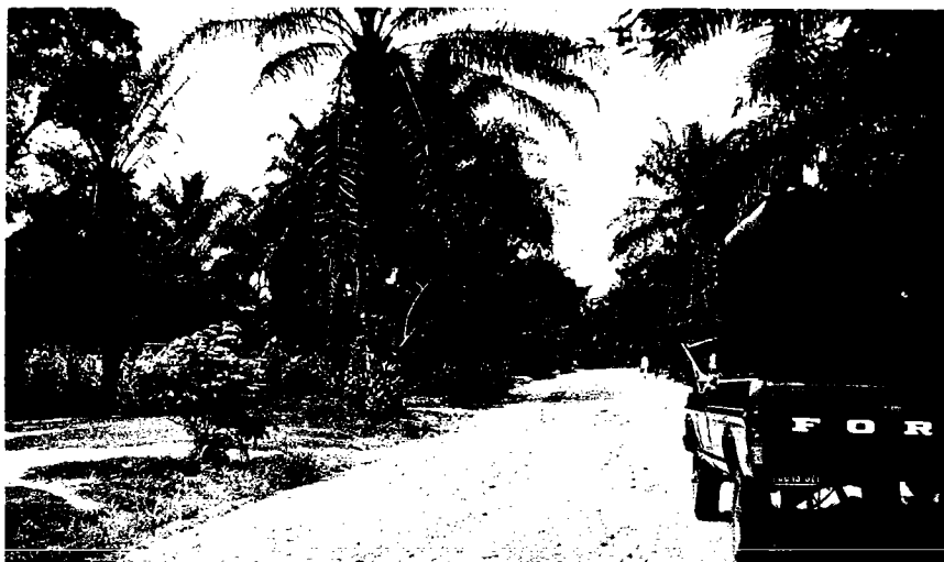
Figure 9. Section of well-maintained road at Bena Mbala on southern alignment. Waste gravels from diamond mining operations are used to surface road.
