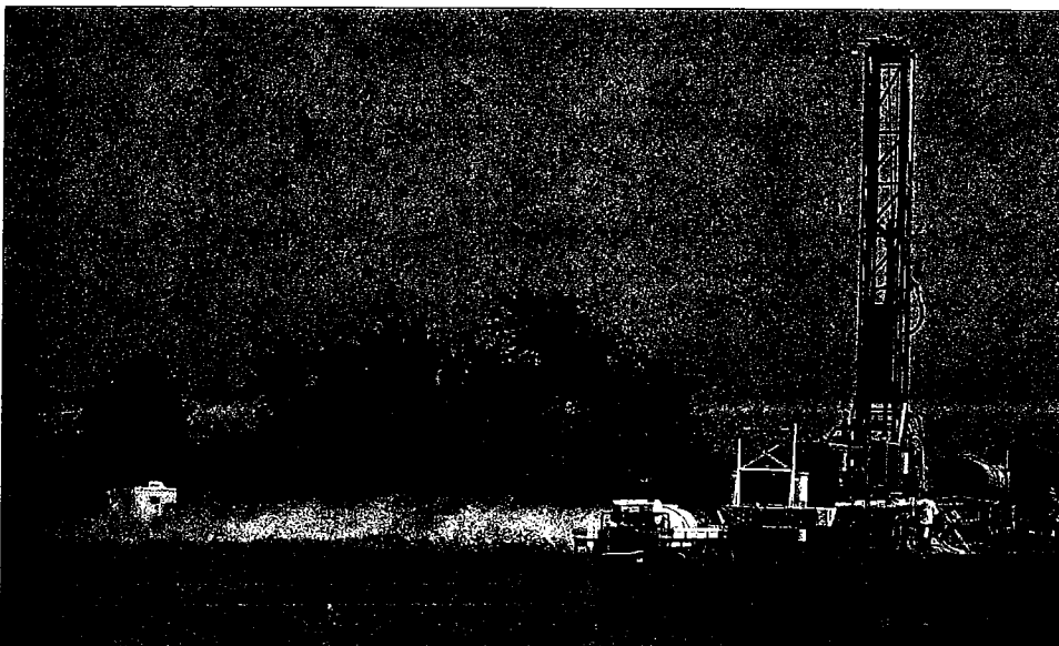
USGS drilling rig at test well. While drilling the deep test hole, air lifted up large volumes of water estimated at up to 1,200 gallons per minute.
