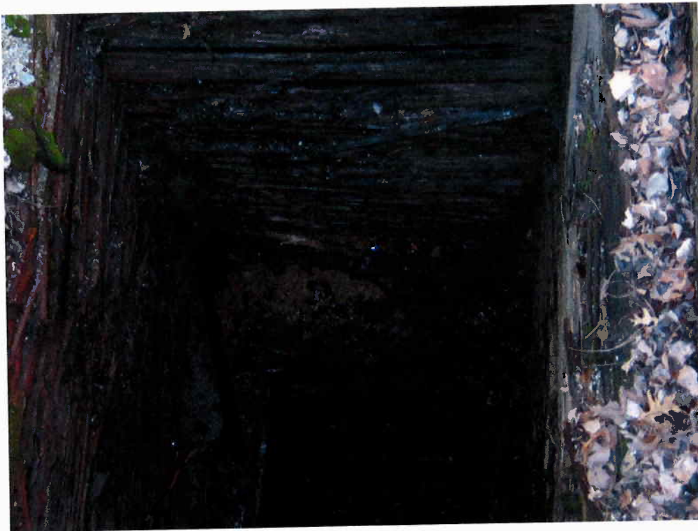
Fig. 1. Open mine shaft on the Cortez lease (T29N, R23E, sec 16, no.12); wooden cribbing still intact.
