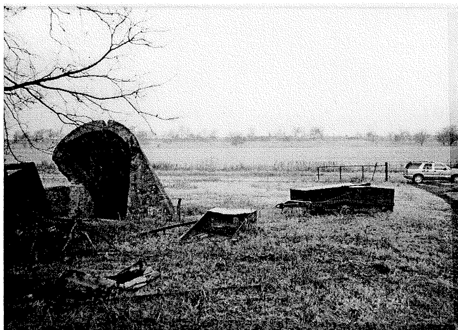
Figure 27. Entrance to Blanco Coal Co. No. 3 mine and rusted machinery. Hendricks (1937a, pl. 2) shows the McAlester coal varying from 2.9 to 3.9 ft thick and dipping 45^{\circ} northwest near here; this is about the same angle as the entrance to the mine.
