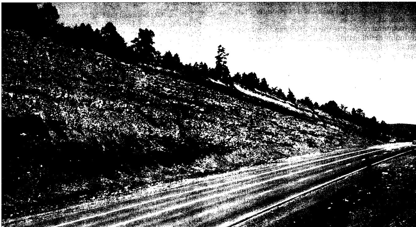
Figure 46. Heavener road cut. Dark-colored strata on left at bottom of outcrop are mostly shales in the Atoka Formation; lighter colored strata above are the lower part of the Hartshorne Formation. Upper Hartshorne sandstone is exposed at the top of road cut, underlain by a conspicuous black band of Lower Hartshorne coal (from Suneson and Hemish, 1994, fig. 68).
