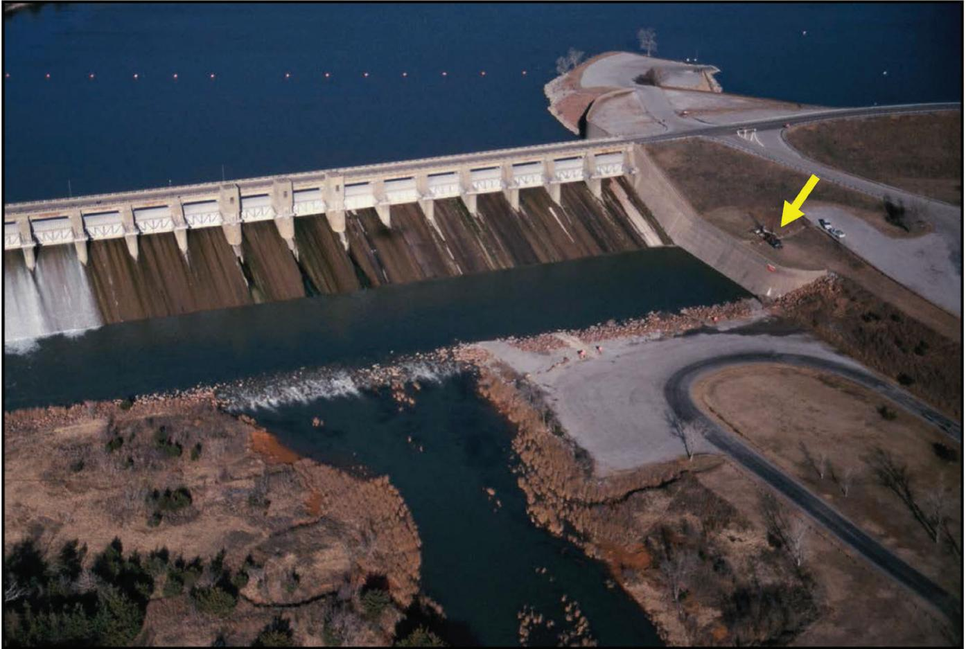
**Figure 4.** Aerial view of primary spillway on Canton Dam, looking north. Also shown is drill rig for borehole BL-2 (arrow) on left spillway abutment, and stilling basin at base of spillway.
