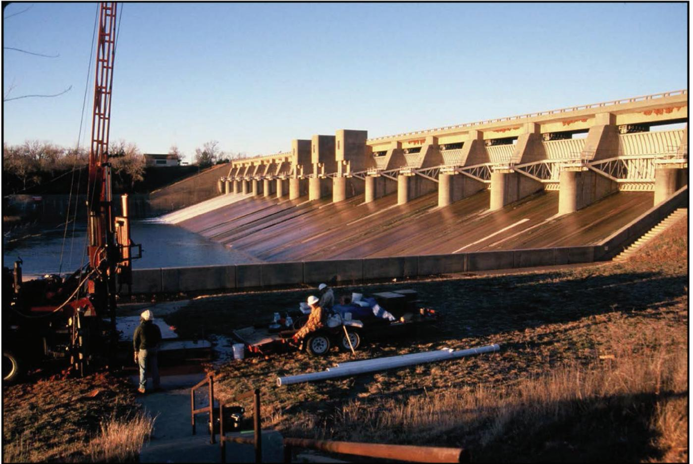
Figure 5. View of primary spillway on Canton Dam and drill rig (on left) for borehole BL-2 on left spillway abutment. View looking to the southwest.
