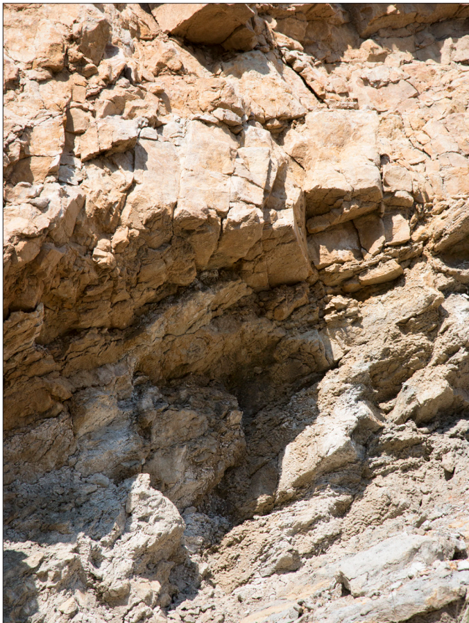
Figure 14. (Left) On the opposite side of I-35 across from the rockfall, blocky more consolidated layers can be seen protruding as ledges over finer-grained material below. The protruding blocks are poised to fall at any time. Figure 15. (Right) Also on the opposite side from the rockfall, vegetation can be seen growing along fractures of the thicker-bedded layers above the finer-grained material. Roots expand the fractures making the rocks more unstable.
