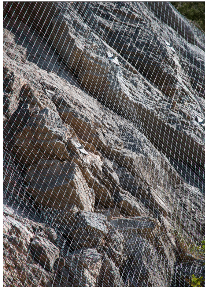
Figure 17. (Above) Bolts were placed in the rock face at the site of the rockfall to provide stability. Figure 18. (Below) A high tensile steel mesh was attached to the rock face to catch rocks that might come unattached.
