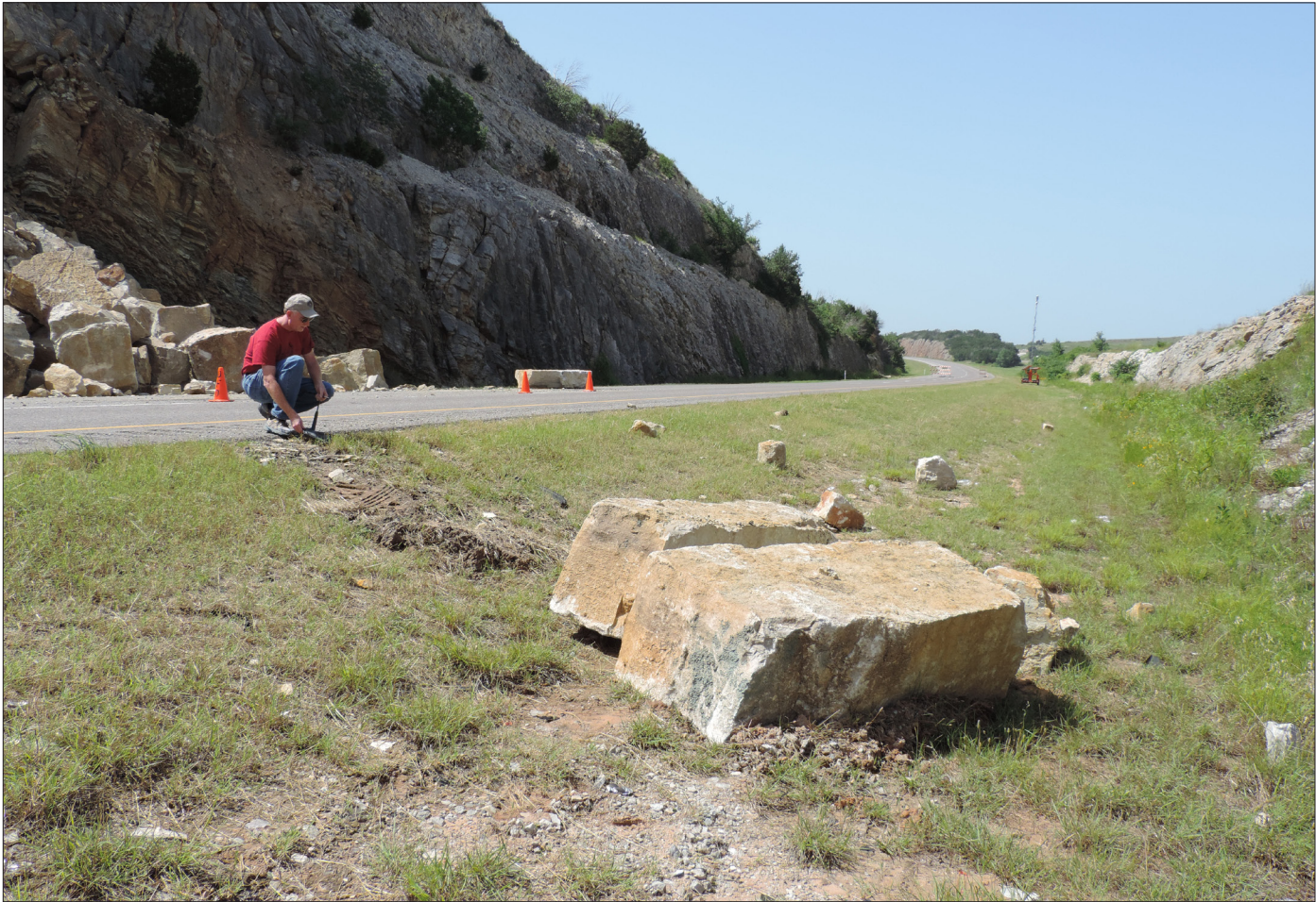
Figure 2. There are various classifications of falling rock and/or soil, which are determined by the materials involved and the way they move from one location to another (Highland and Bobrowsky, 2008; Stock and others, 2013). Because the rocks in this case were thought to have broken free and fallen down the slope, the incident is being termed a rockfall. Note the northbound lanes of I-35 were closed for six weeks to allow for debris removal and safety enhancements.
