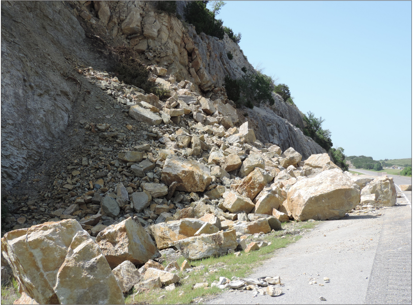
Figure 9: A fan of rock debris lays scattered along the side of the road, with large rocks falling onto the road.
