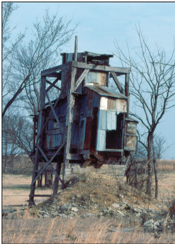
Figure 5. Derrick used by a two- to four-man crew to gain access to an underground mine, the Blacksnake. These crews were called 'gougers' by the local people.
