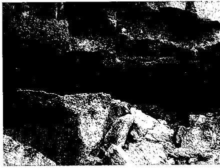
Figure 3. Fracture surfaces in the rock ledge above the entrance to Alabaster Cavern after the collapse had occurred.
