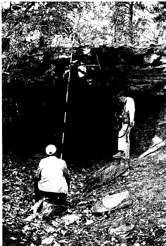
Figure 14. Portal (Le Flore County)—a surface entrance to a mine drift, tunnel, adit, or entry that is not sealed or barricaded. It poses a threat when it is located close to a populated area, public road, or other area of intense visitation.
