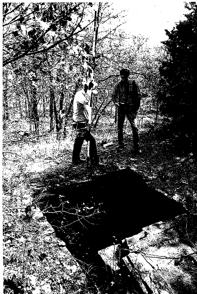
Figure 15. Vertical opening (Le Flore County)—[1] a vertical or steeply inclined mine shaft or opening that is not sealed or barricaded, or [2] a hazardous vertical opening to a mine caused by subsidence (see Fig. 10A). Such an opening is considered a threat to the public whether or not it is close to a populated area, a public road, or other area of intense visitation.
