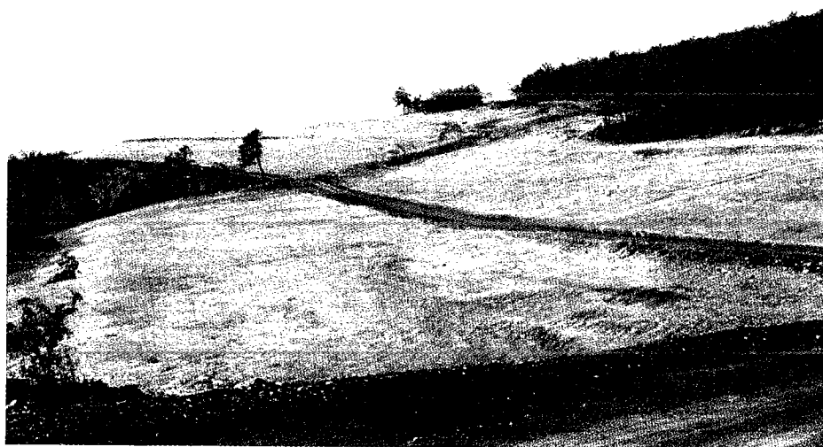
View looking southwest of recent reclamation in the Georges Colliers, Inc., Pollyanna No. 6 coal mine on the east side of Cavanal Mountain (sec. 22, T. 7 N., R. 27 E.) in north-central Le Flore County, Oklahoma. The medium-volatile bituminous Secor coal (Boggy Formation; Desmoinesian) was mined to a maximum depth of 85 ft from 1990 through 2000.
