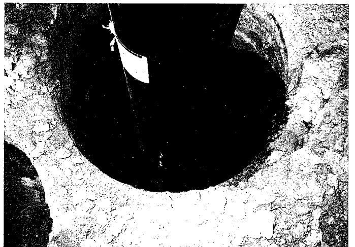
Figure 11. Water seeping into a hole drilled for footings for playground equipment being installed on church property, July 1999.
