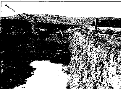
Figure 16. Wister coal mine in Le Flore County, with dragline, head-wall, and drill rig used for drilling shot-holes. This mine is typical of Oklahoma strip mines.
