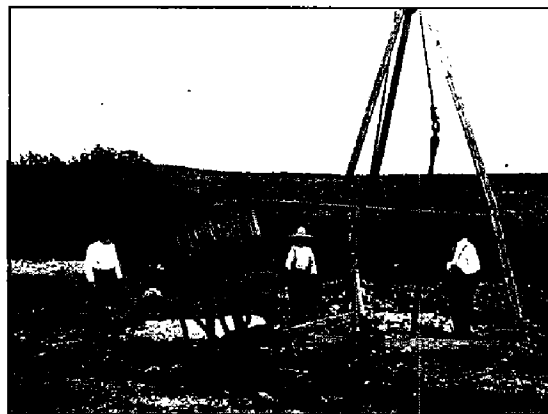
Figure 23. Cable-tool rig used to explore for zinc in the Southwest Davis zinc field. Gertrude Sober in center. Photo taken in 1909.
