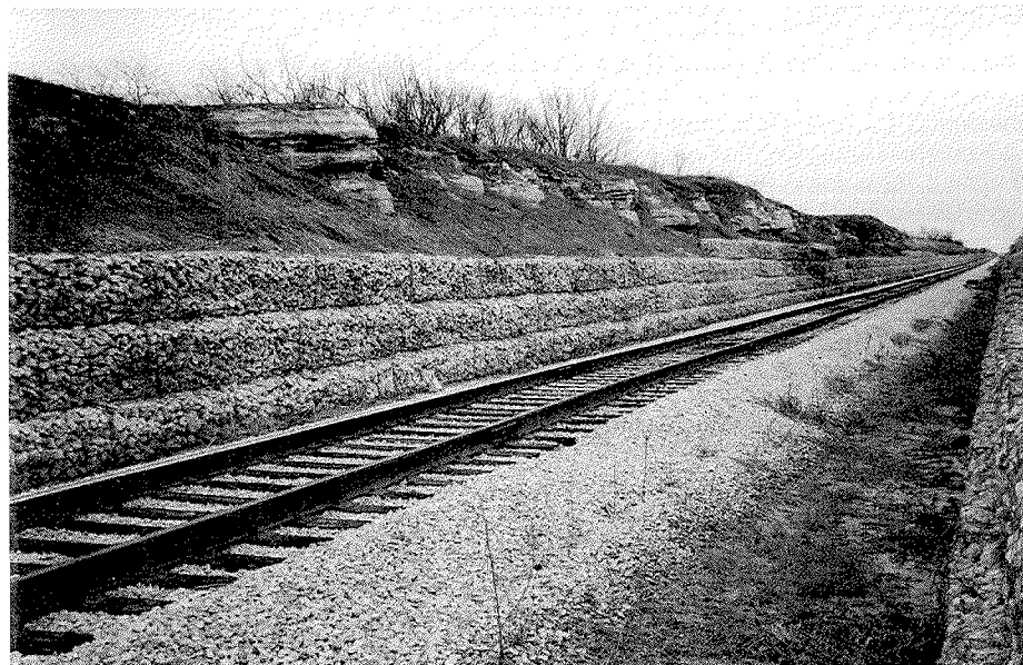
Figure 9. Riprap consisting of crushed limestone is confined in heavy-gauge wire mesh along this cut, nearly 0.25 mi long, in the NW¼ sec. 17, T. 22 N., R. 16 E. The riprap prevents erosion of shales in the Lagonda Sandstone Member of the Senora Formation. The light colored, resistant rock at the top of the cut is the Breezy Hill Limestone, underlain by a covered interval containing the Kinnison Shale and Iron Post coal.
