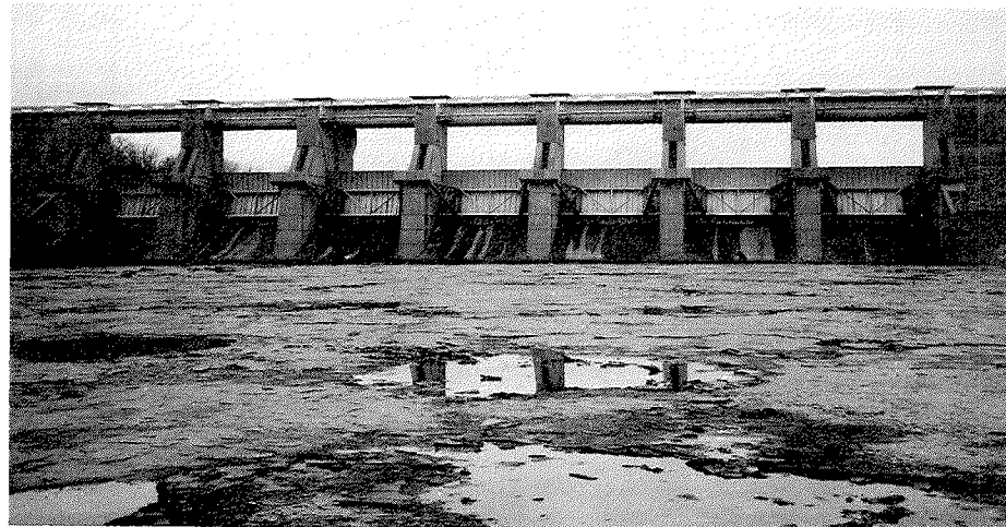
Figure 4. The Oologah Lake spillway showing the floodgates. S.H. 88 bridge crosses the structure (at top).
