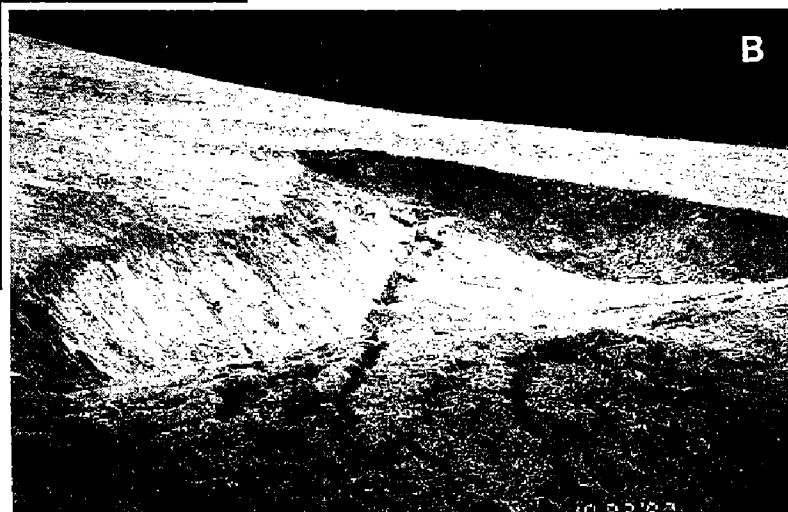
Figure 7. A—Slump on graded slope in Sans Bois Mountains along new segment of S.H. 82. B—Close-up view of same slump scar from the opposite side. Photographed by C. J. Hayes, ODOT, October 23, 1997.
