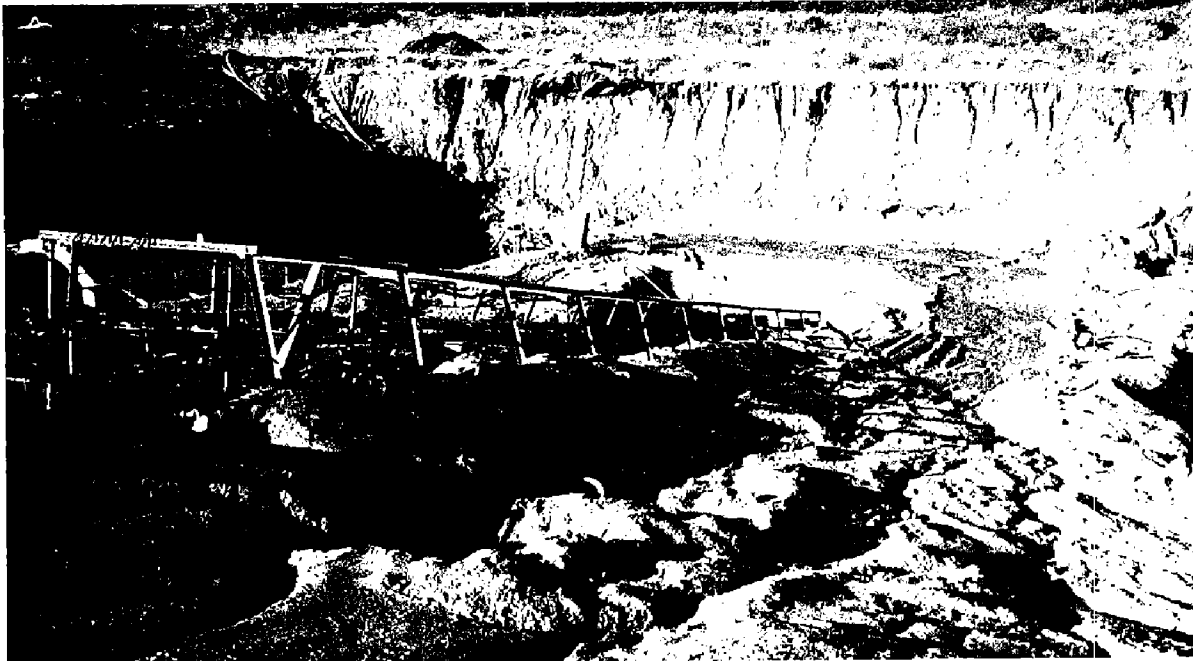
Figure 2. Highwall of the pit excavated prior to digging the entry tunnels for the slope mine. The conveyor system used to bring coal from the mine is shown emerging from the center entry.
