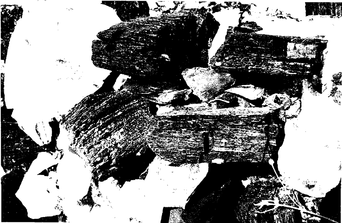
Figure 4. Bright-banded coal and glass cullets in phase 1 retaining wall along back of house, showing loss of luster, lack of contrast between bands, and deep fractures.
