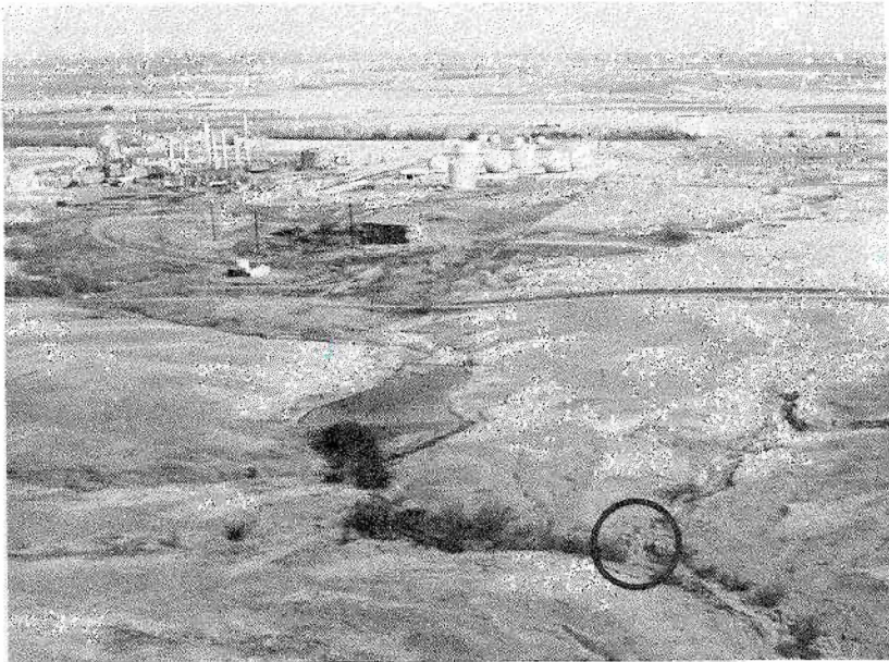
Figure 8. Oblique aerial view of blowout site (crater circled), looking north-west, with Shell Oil Company natural-gas-processing plant in background. White building north of section-line road extending across photograph just above center marks location of 1-SWD Yelton well, and lone tank south of the six tanks is salt-water-storage tank for 1-LPG Yelton well, directly to west.
