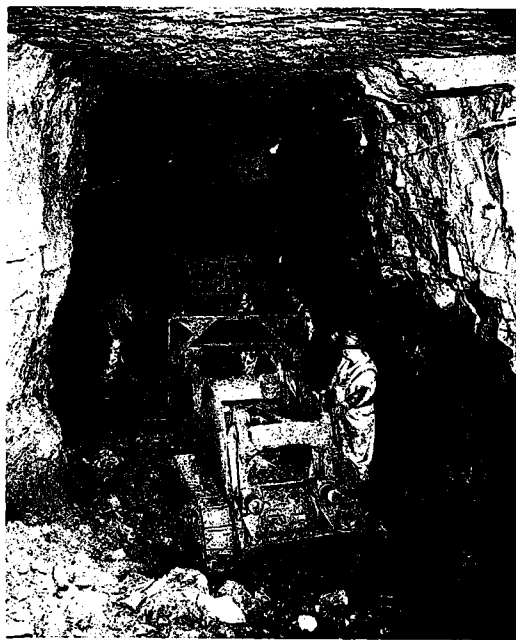
Figure 4. Photograph of underground operations with a view of the mine shaft in the background and showing 4-foot shale stratum in Wreford Limestone.
