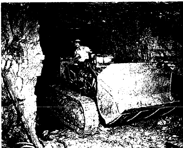
Figure 5. Photograph showing calcareous siltstone in Wreford Limestone in tunnel of Continental Oil Company's underground storage cavern near Ponca City. (Photograph courtesy of Continental Oil Company)
