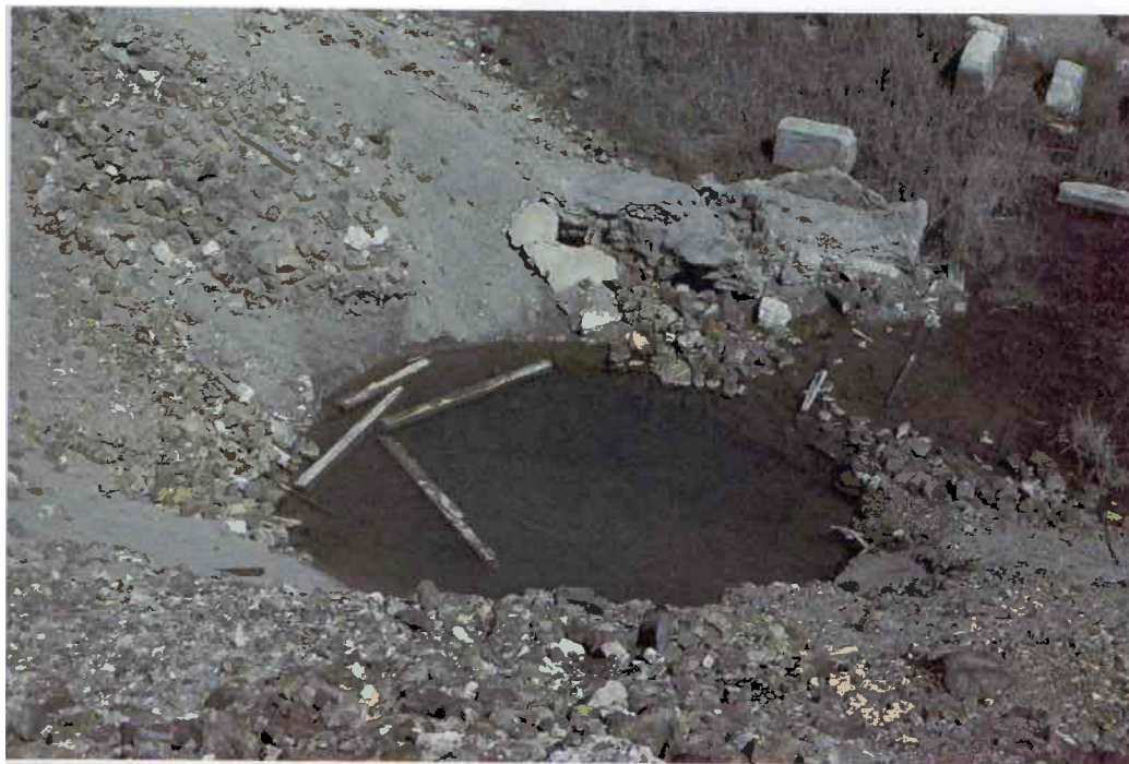
Figure 11. A 20-ft-diameter circular collapse, Howe Mine, 29N-23E-17(41).
