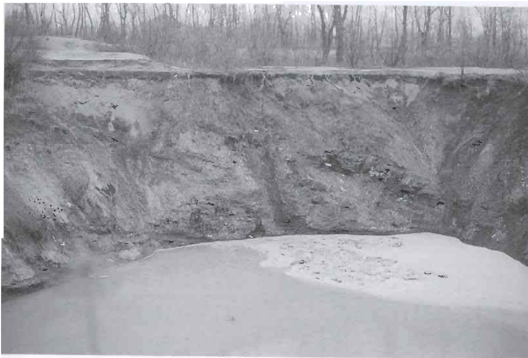
Figure 18. A 240- × 160-ft elliptical non-shaft collapse, Crystal Mine, 29N-23E-19(1504); water level is 45 ft from surface.
