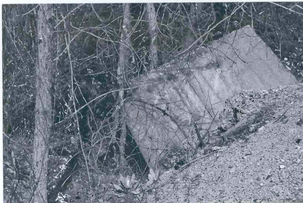
Figure 14. A 6.5-ft concrete cube used to seal a shaft on Grace Walker lease, 29N-23E-21(41).
