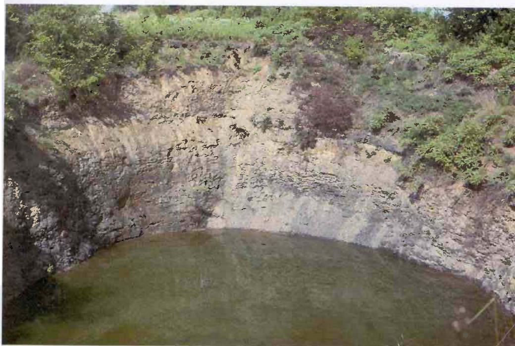
Figure 12. A 180- x 100-ft elliptical collapse, Gordon No. 2 Mine, 29-23E-18(8). Water level is approximately 35 ft below surface.
