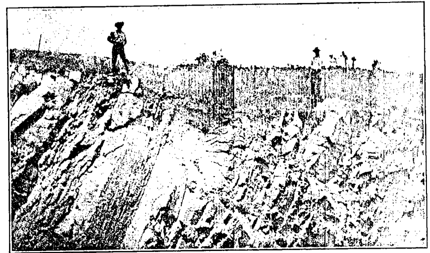
A. The outcropping edges of two resistant, siliceous, limestone beds with 12 feet of sandy shaly limestones between illustrating how the thin beds weather and become covered with vegetation. About 500 feet below the top of the Arbuckle along Ardmore-Davis road.
