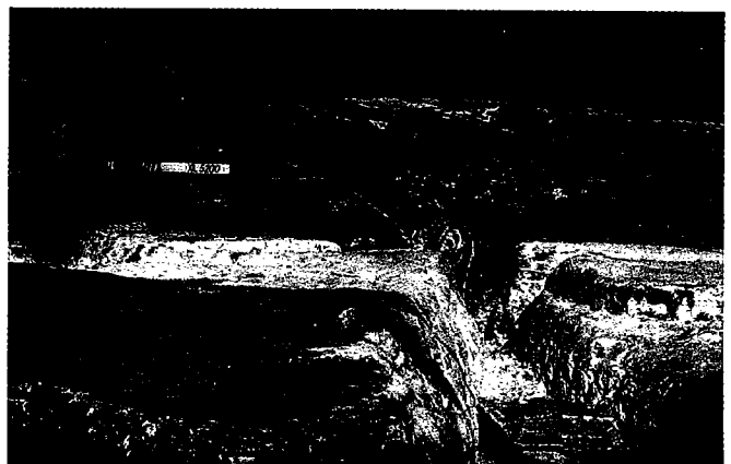
Figure 14. Final surface preparation by cleaning clay from solution-enlarged fractures at Fort Dodge, Iowa.
