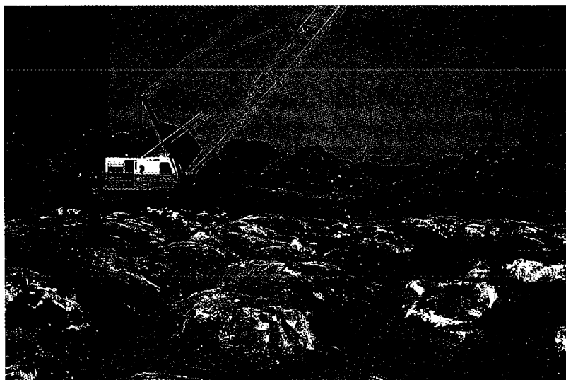
Figure 12. Cleaning of hummocky bedrock surface of gypsum by dragline at Sweetwater, Texas.
