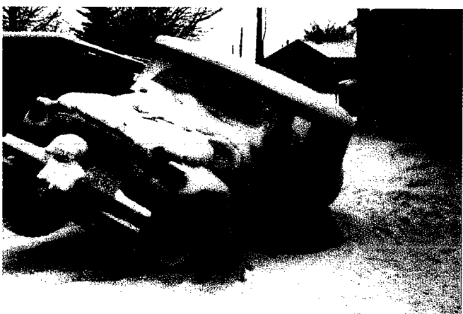
Figure 10. Sudden collapse in alley caused by piping in the underlying gypsite, Laramie. Foster White photo.
