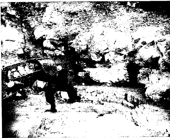
Figure 10. Solution-enhanced fractures in dolomite of the Tensleep Formation in the north abutment of Anchor Dam. Reproduced from U.S. Bureau of Reclamation (1962).
