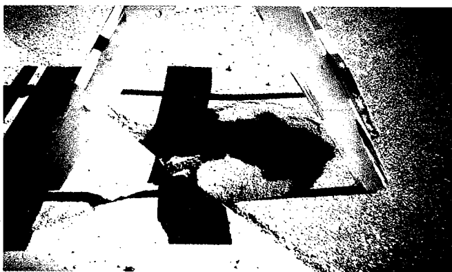
Figure 9. Collapse of asphalt next to a seam between a concrete gutter and the asphalt pavement owing to dissolution of the underlying gypsite, Laramie. Foster White photo.
