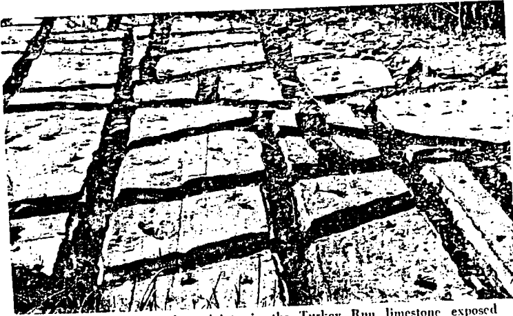
Figure 16. Solution along joints in the Turkey Run limestone exposed in the bed of Hellroaring Creek just east of the fault in SE \frac{1}{4} sec. 6, T. 21 N., R. 7 E., looking southeast.
