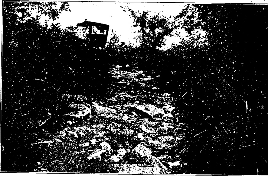
Fig. 42. Natural Roadway over Limestone near Hardy.
