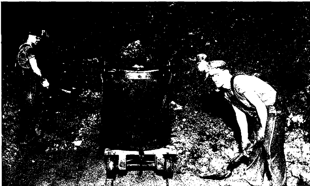
B. Shovelling crude ore into buckets
