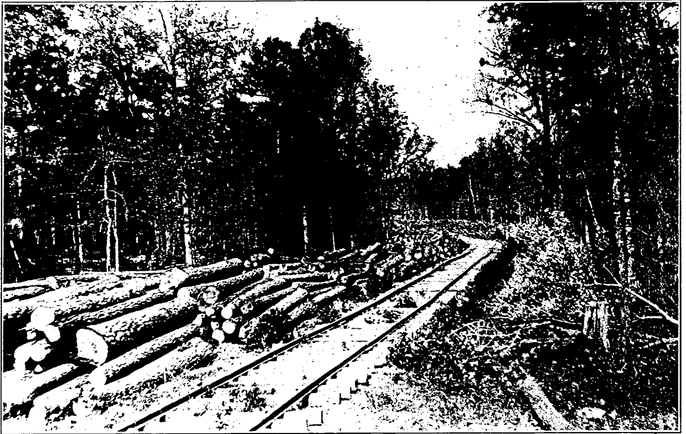
TEMPORARY TRAMWAY, SEC. 10, T. 4 S., R. 20 E., CONSTRUCTED FOR THE PURPOSE OF HAULING OUT THE PINE LOGS.
